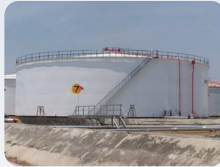
BBM Storage Tank- Blue Sky Project Pertamina UP VI Balongan Indramayu
