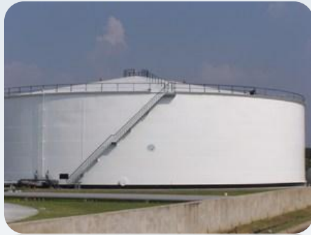
BBM Storage Tank Depot Plumpang Pertamina UPMS III Jakarta
