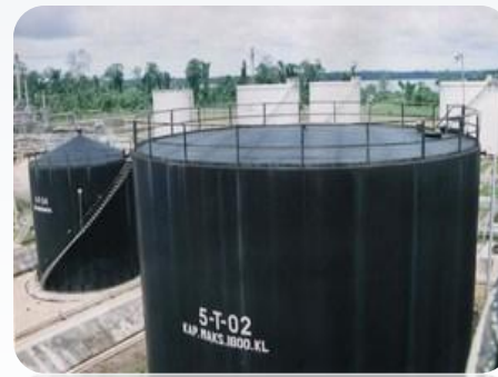
BBM Storage Tank- Pertamina UP Sorong Papua
