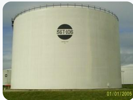
BBM Storage Tank Pertamina UP IV Cilacap - Jawa tengah
