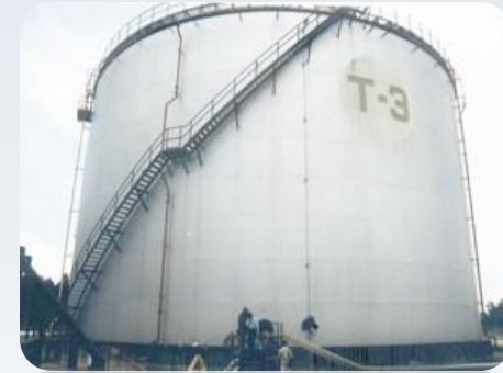
Avtur Storage Tank Pertamina UP VI Ambon
