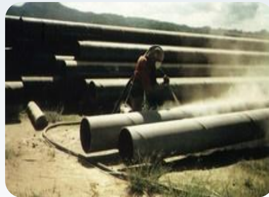
Pipeline BBM Pertamina UP VI Ambon
