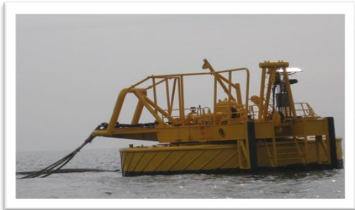
Single Mooring Bouy PT. Pertamina Balongan 2009
