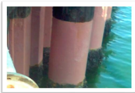
Tiang Pancang Dermaga PT. Kaltim Methanol Industri 2008
