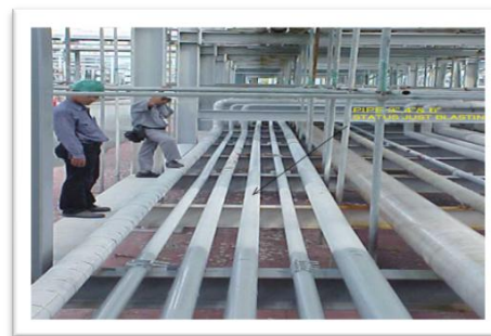
Struture Pipe Rack PT. Badak NGL - Kaltim 2005-2006
