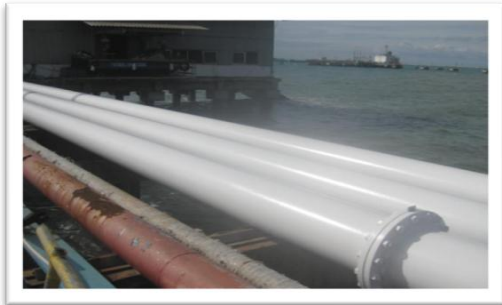
BBM Line Pipe PT. Pertamina Tj. Gerem - Cilegon 2009
