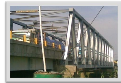
Jembatan Eretan PU Bina Marga - 2008 Epoxy (75 micron) - Acrylic (50 micron) Simacover EP Unicoat - Simacare Finish
