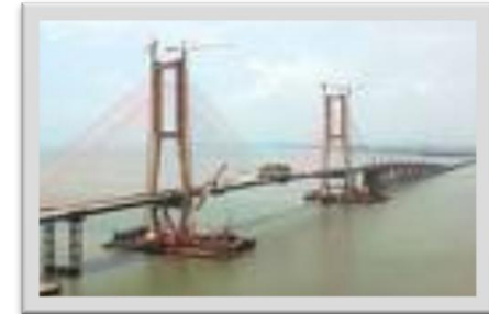
Jembatan Suramadu PU Bina Marga - 2004 Epoxy (75 micron) - Polyurethane (75 micron) Simacover EP Unicoat - Simathane Gloss
