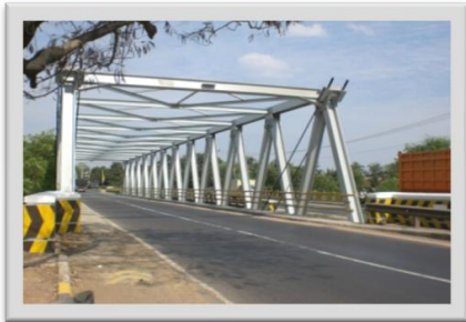
Jembatan Balonggandu PU Bina Marga - 2007 Epoxy (75 micron) - Acrylic (50 micron) Simacover EP Unicoat - Simacare Finish
