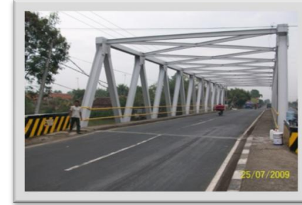
Jembatan Kalimenir PU Bina Marga - 2009 Epoxy (75 micron) - Acrylic (50 micron) Simacover EP Unicoat - Simacare Finish
