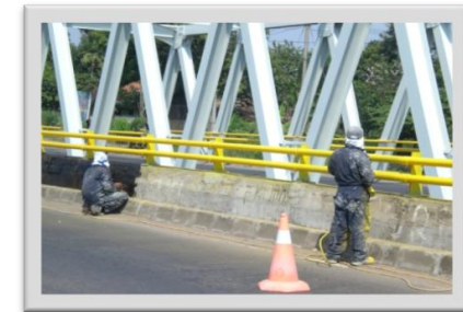
Jembatan Gintung PU Bina Marga - 2009 Epoxy (75 micron) - Acrylic (50 micron) Simacover EP Unicoat - Simacare Finish
