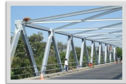
Jembatan Sewo PU Bina Marga - 2009 Epoxy (75 micron) - Acrylic (50 micron) Simacover EP Unicoat - Simacare Finish
