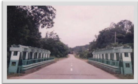
Jembatan Batang Lolo 3 PU Bina Marga - 1999 Epoxy (75 micron) - Polyurethane (75 micron) Simacover EP Unicoat - Simathane Gloss
