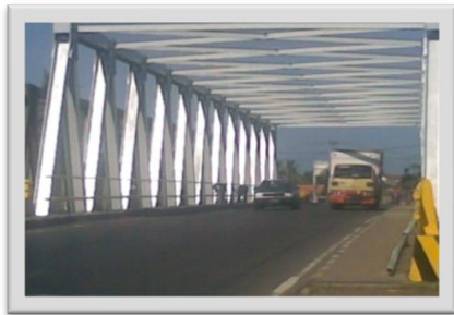
Jembatan Cipunegara PU Bina Marga - 2008 Epoxy (75 micron) - Acrylic (50 micron) Simacover EP Unicoat - Simacare Finish
