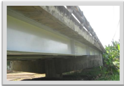
Jembatan Kenanga PU Bina Marga - 2009 Epoxy (75 micron) - Acrylic (50 micron) Simacover EP Unicoat - Simacare Finish
