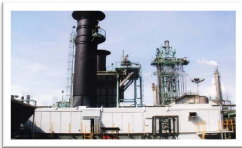
Cerobong PT. PUSRI 2004
